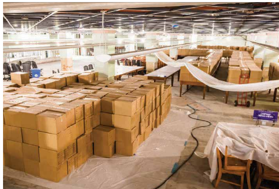
Soot-covered furniture and boxes of books await removal from Hale Library's first floor. Most tables and chairs suffered smoke damage and were unsalvageable.
