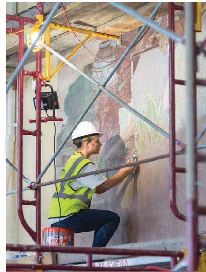
In fragile areas, a thermoplastic adhesive was injected into the murals and then heated to keep the paint from flaking off of the wall.
