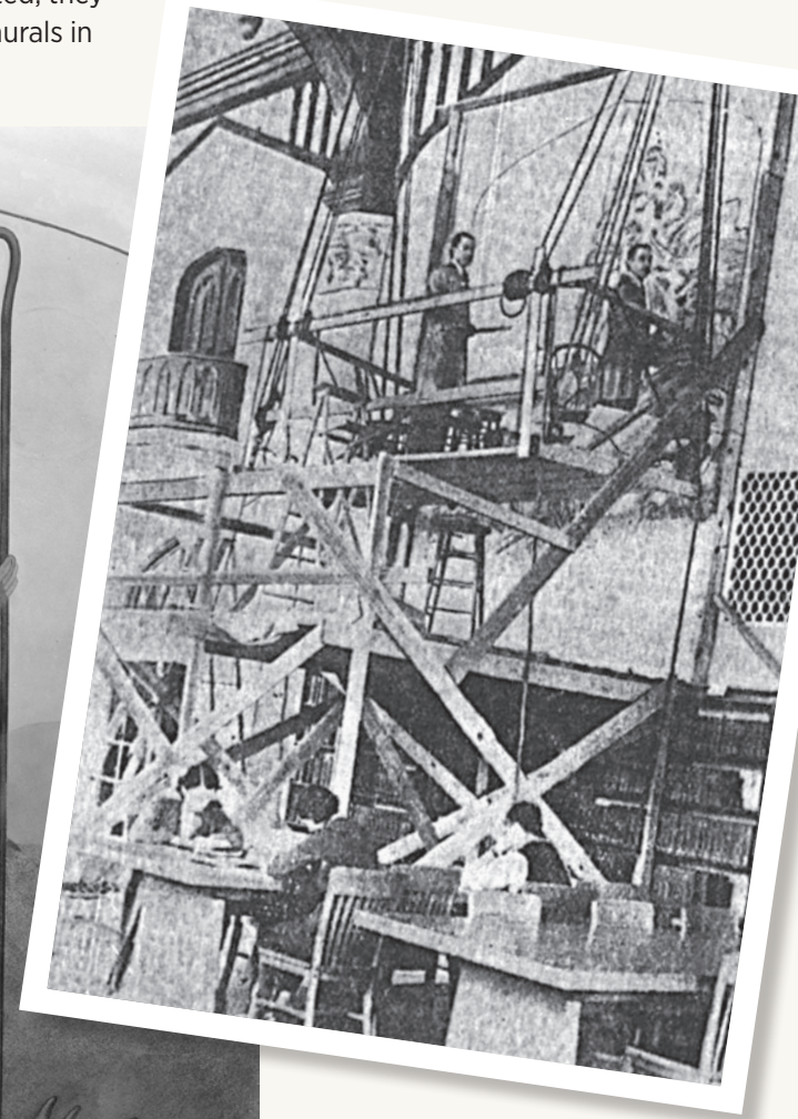
Above: Overmyer (right) and Wolfe (left) using scaffolding and materials supplied by K-State.
